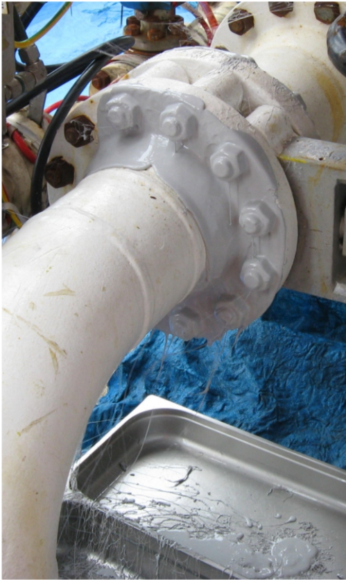
Application builds coats in succession, working from underneath, around the sides and finally above with two coats to provide maximum protection. The underside is the most difficult area to finish aesthetically but trimming between and after each coat ensures full protection. All trimmings and drips/spills are collected and recycled.
