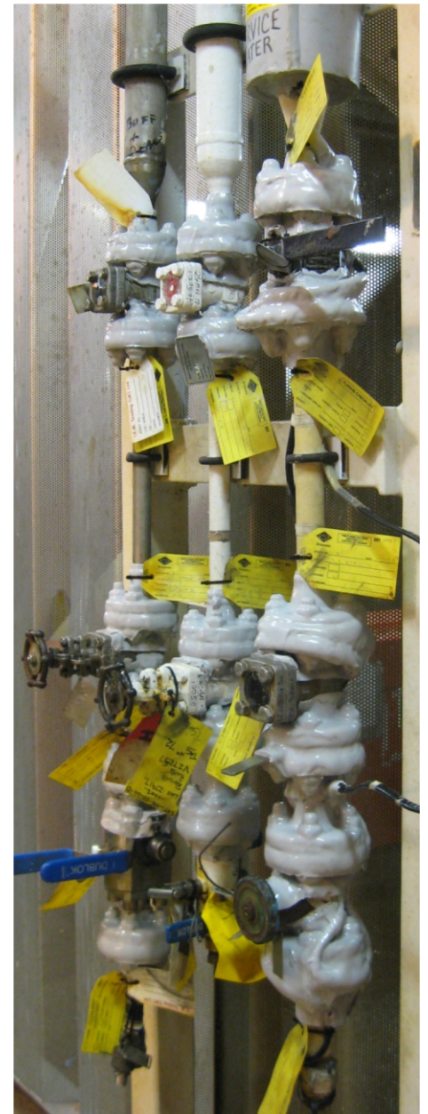
Below: during application a joint can look messy, but once both coats are completed and trimmed the joints look, and are, ready for the worst conditions the North Sea can throw at them!
