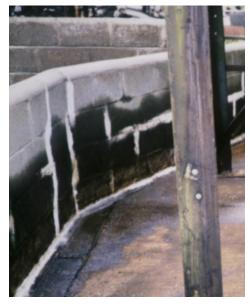
possible but, as the photo below shows, much remained both on and below the surface. Cracks and joints were repaired and then a sealing coat of Alocit 28.95 was applied followed by a finishing coat of Alocit 28.15 in standard gray.
